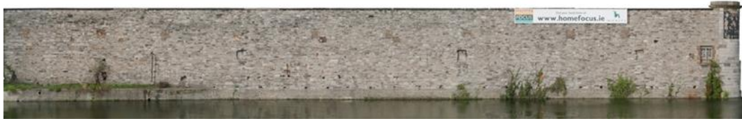
Figure 12.12: Riverside Stone Wall
